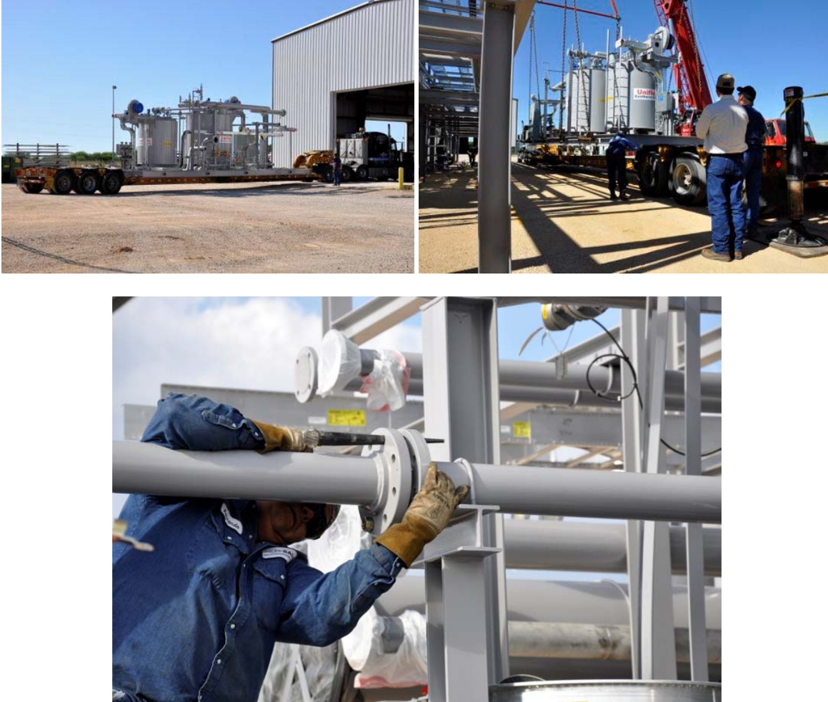
Figure 16: Transporting, rigging, and aligning module to module connections.
