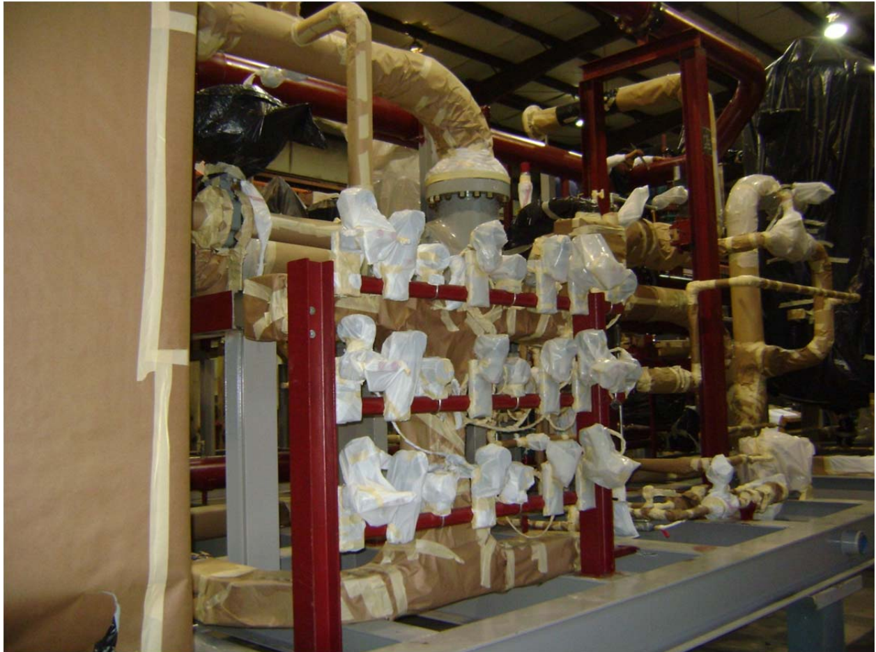
Figure 15: The process module is "taped off" and ready for paint.
