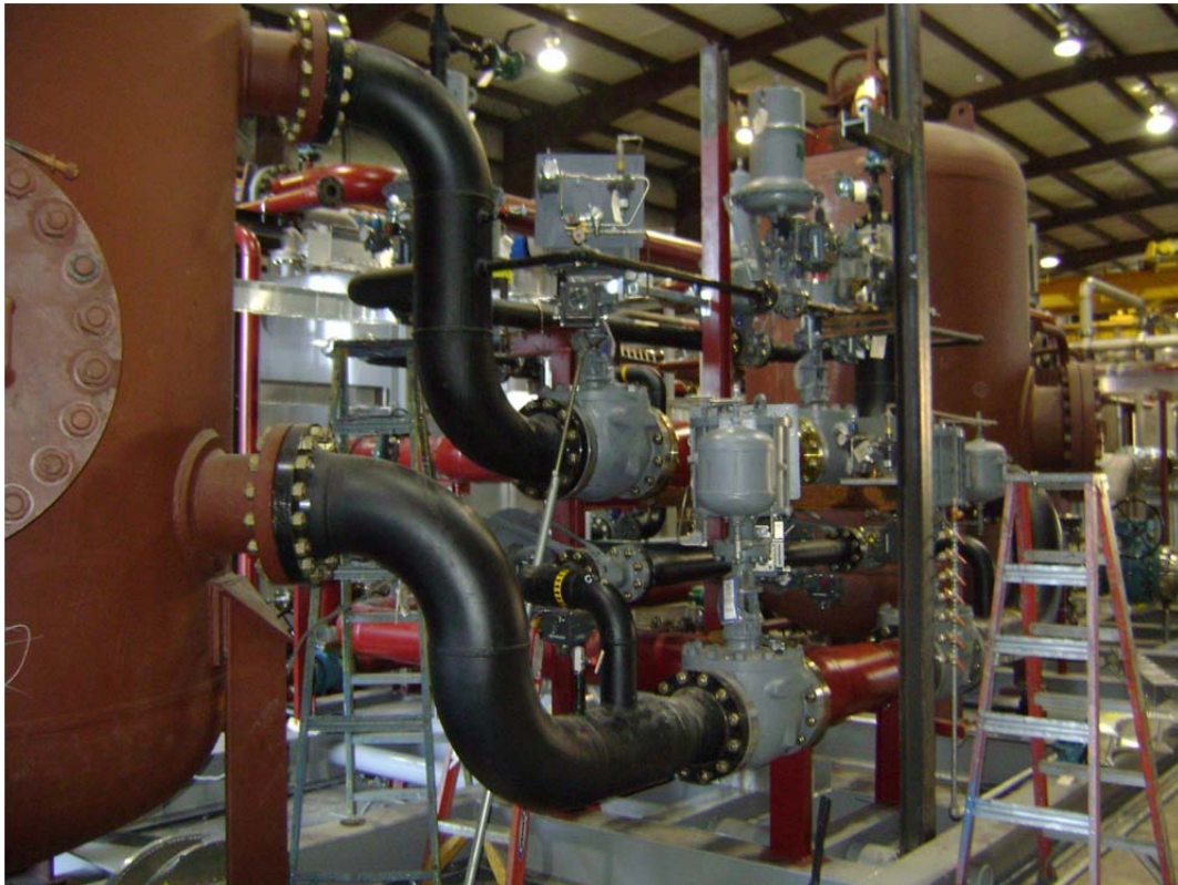
Figure 6: Piping spools installed and ready for pressure testing.
