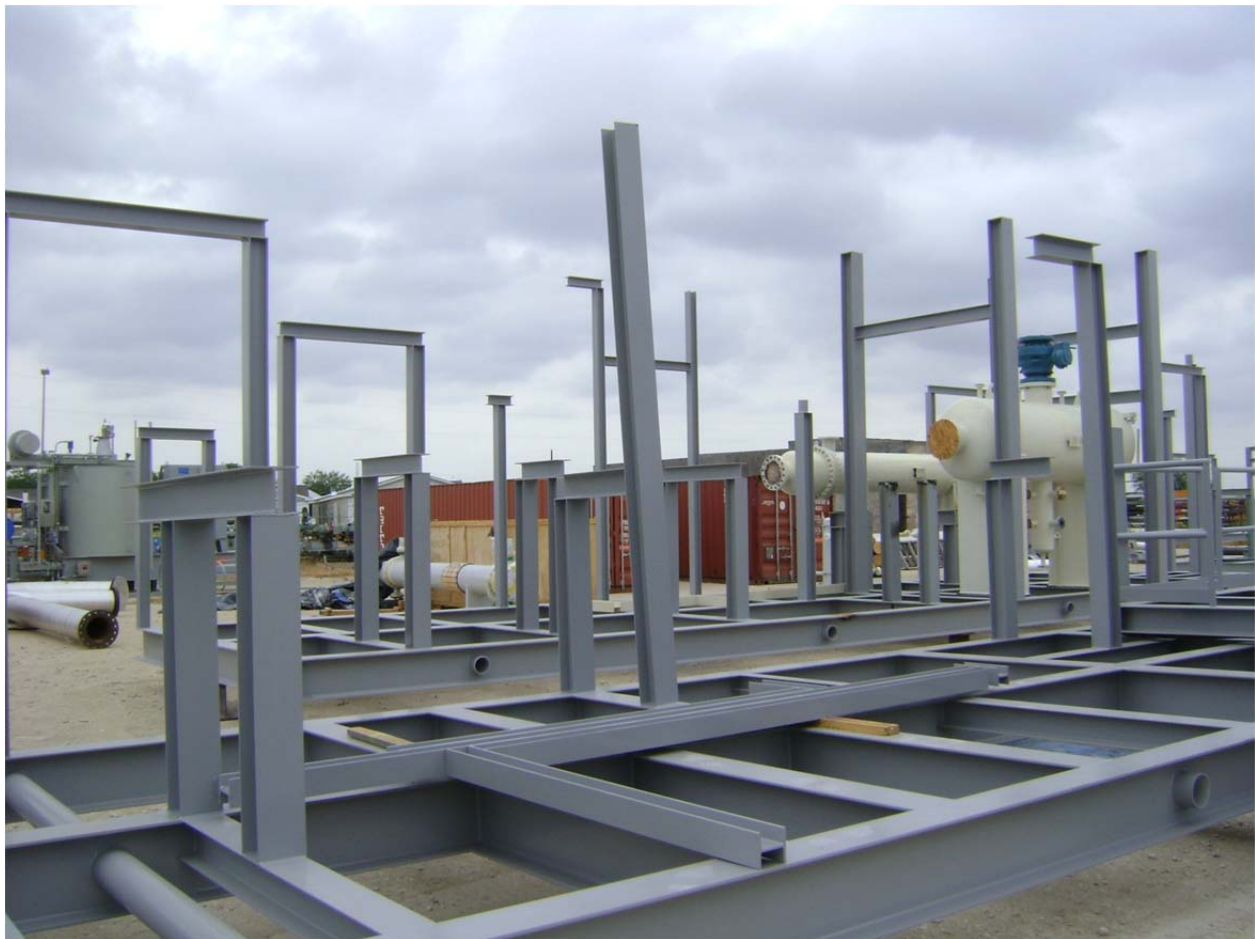
Figure 3: Skid steel is the first phase of the modular manufacturing process
