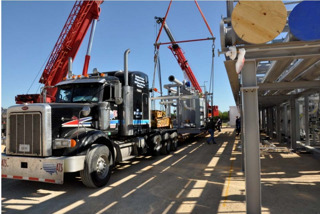
Figure 20: Qualified Crane and rigging teams offload process modules into position
