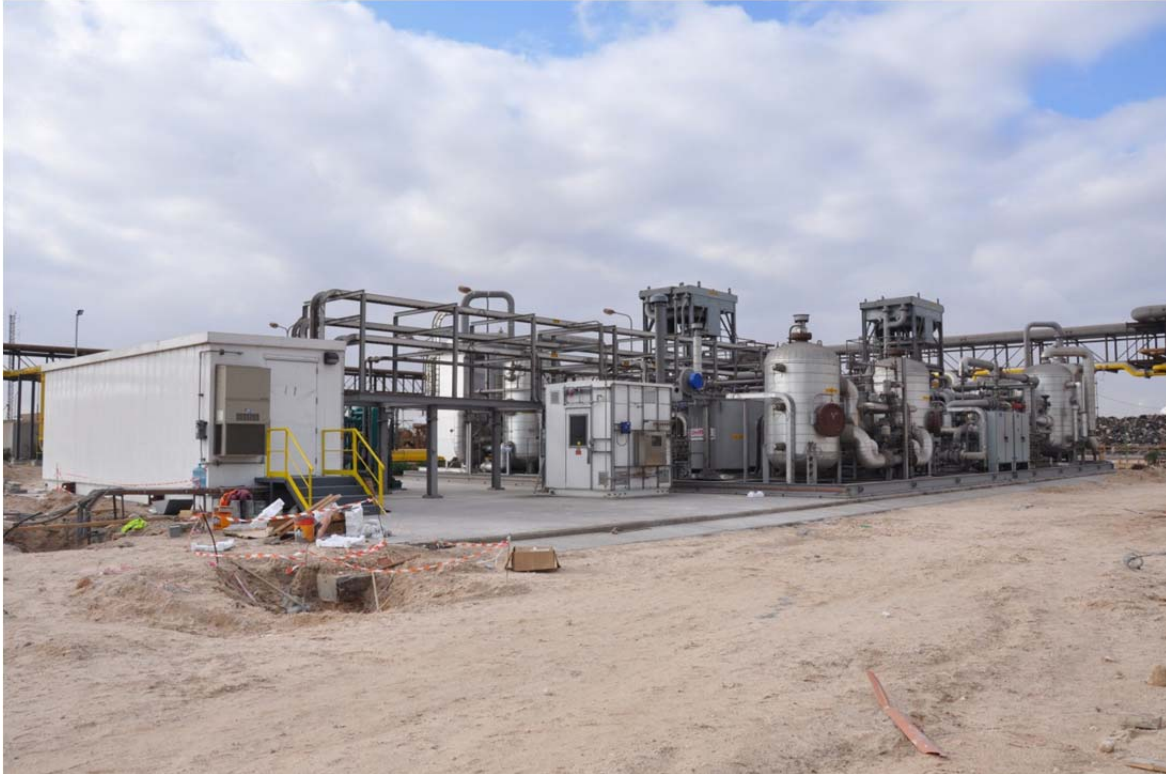
Figure 25: On site assembled.
