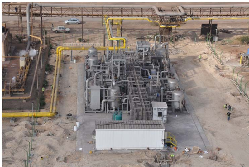
Figure 23: Permanently installed at the customer location.
