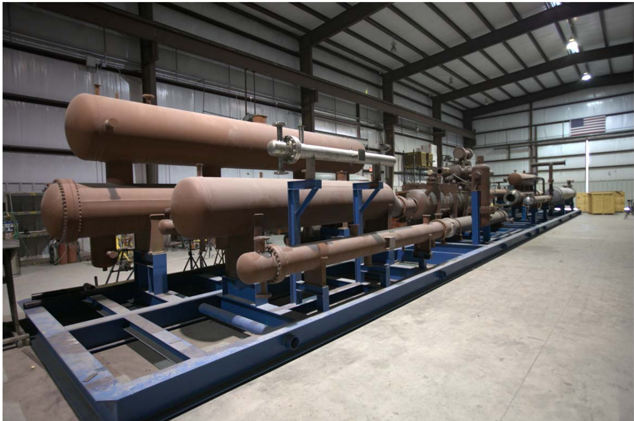
Figure 4: Major equipment set in place.
