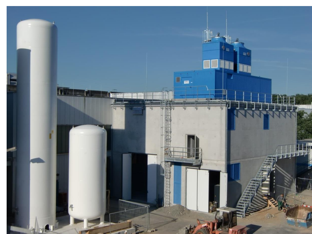
Annex building with 100 m³ and 50 m³ Helium Tanks
